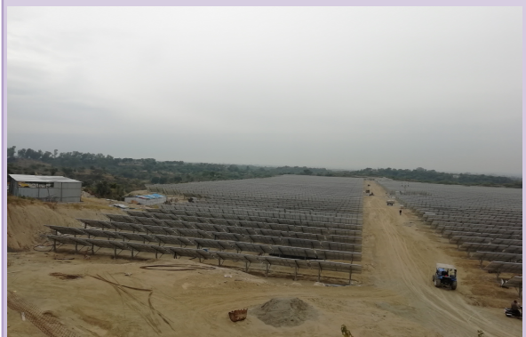
Bera Dol Solar Power Plant
