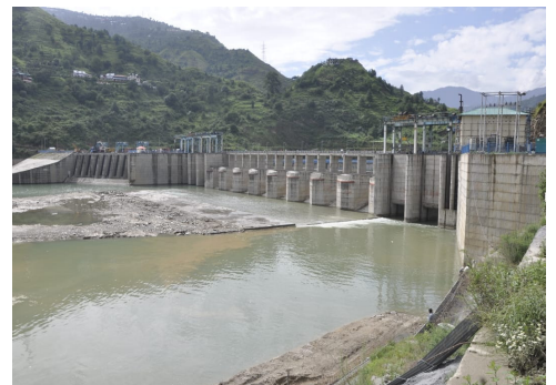
Barrage of 111 MW Sawra Kuddu Hydro Electric Project
