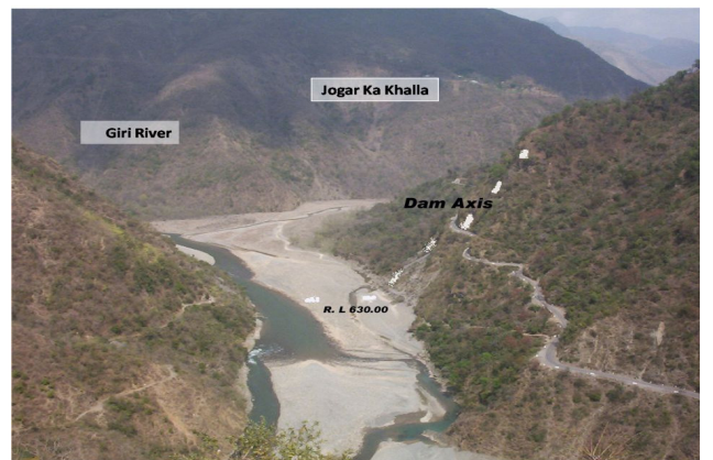
Site of Renukaji Dam Project
