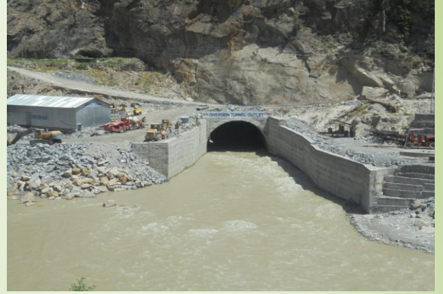
Diversion Tunnel Outlet of Shongtong Karchham HEP
