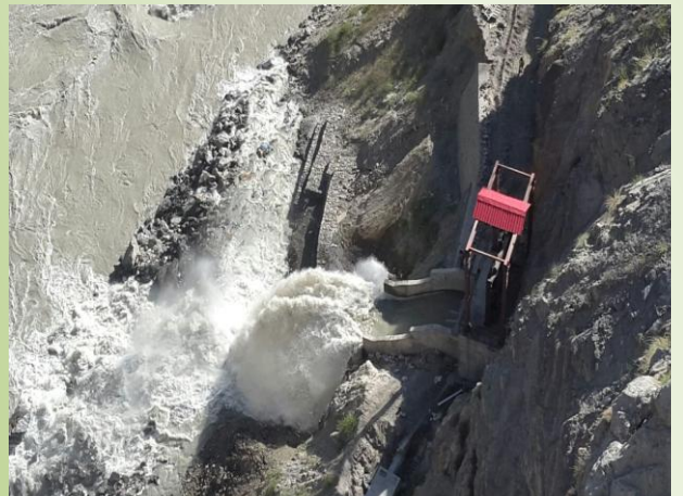
Outfall of Kashang HEP
