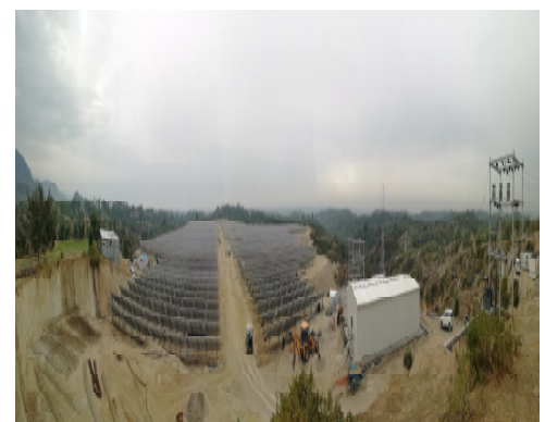
View of 5 MW Berra Dol Solar Power Project
