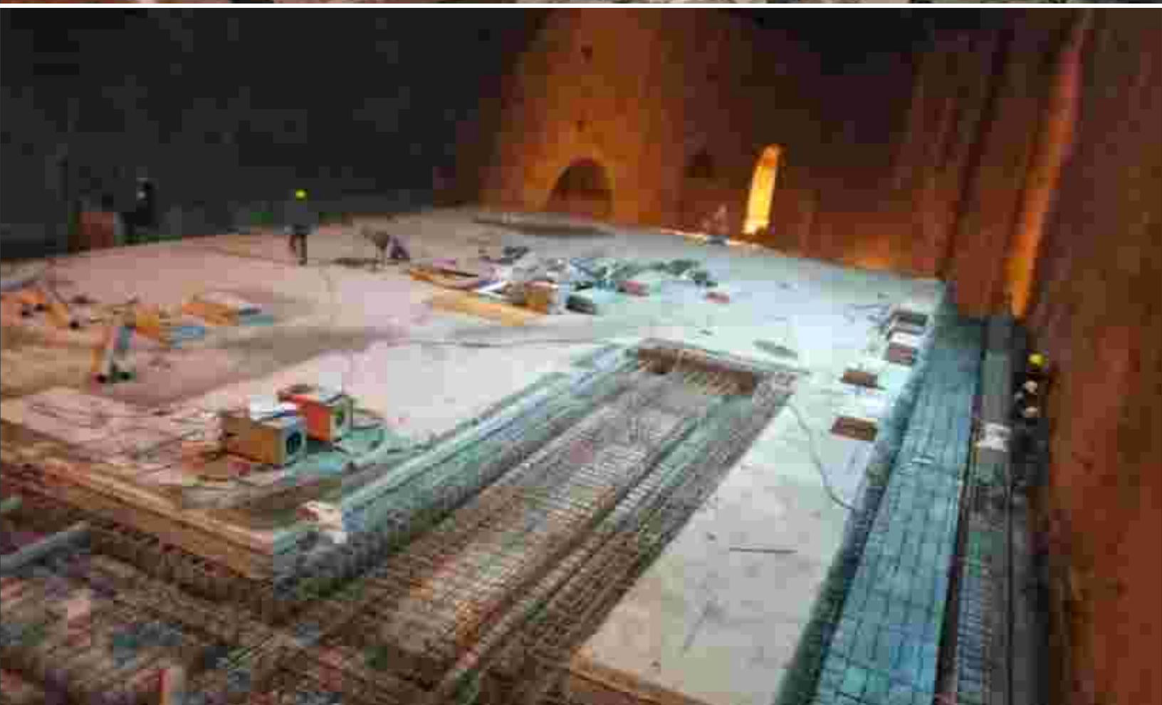
Service Bay Concreting in Progress, Shongtong Karcham HEP (450 MW)
