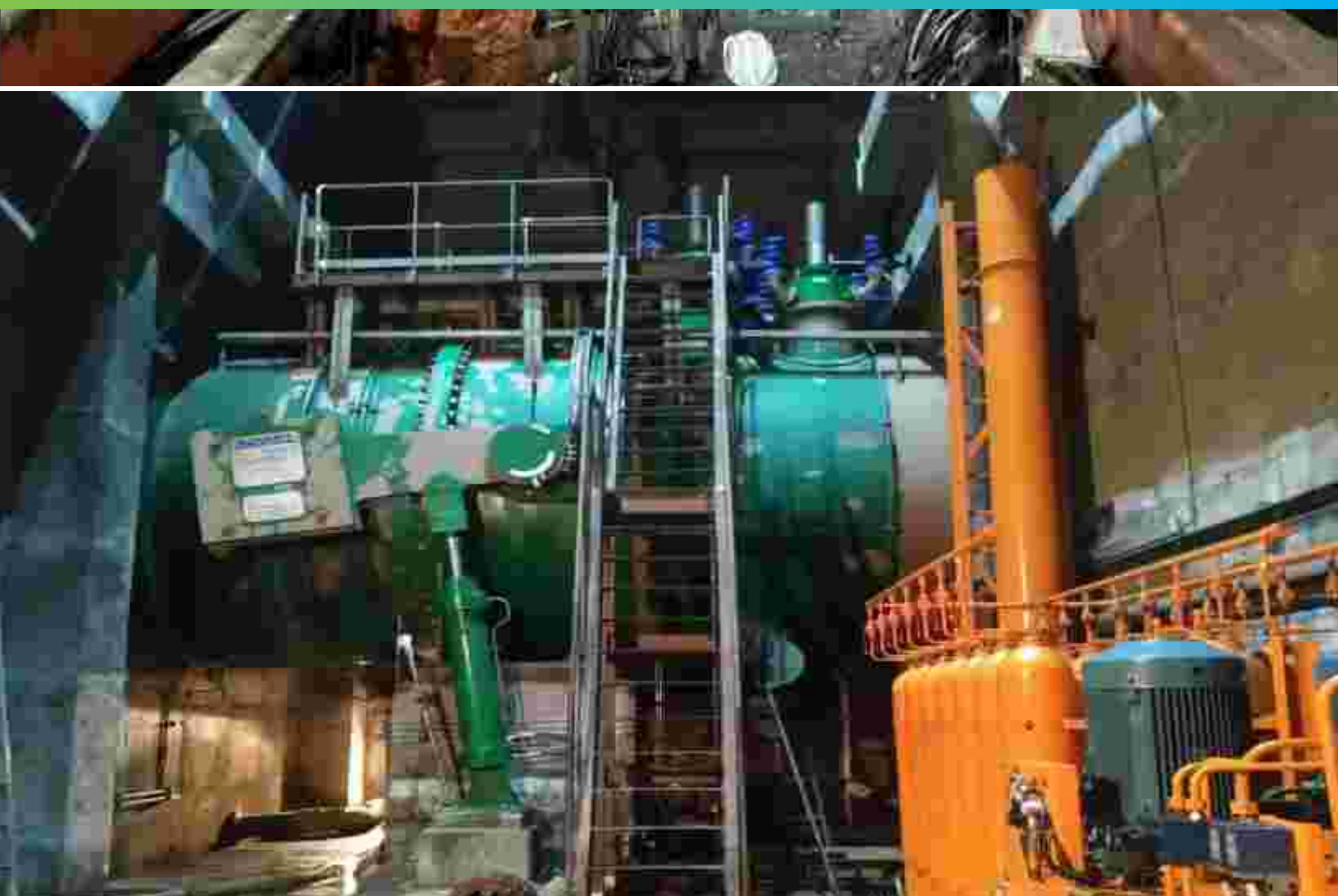
Main Inlet Valve, Sawra Kuddu HEP (111 MW) PH Package
