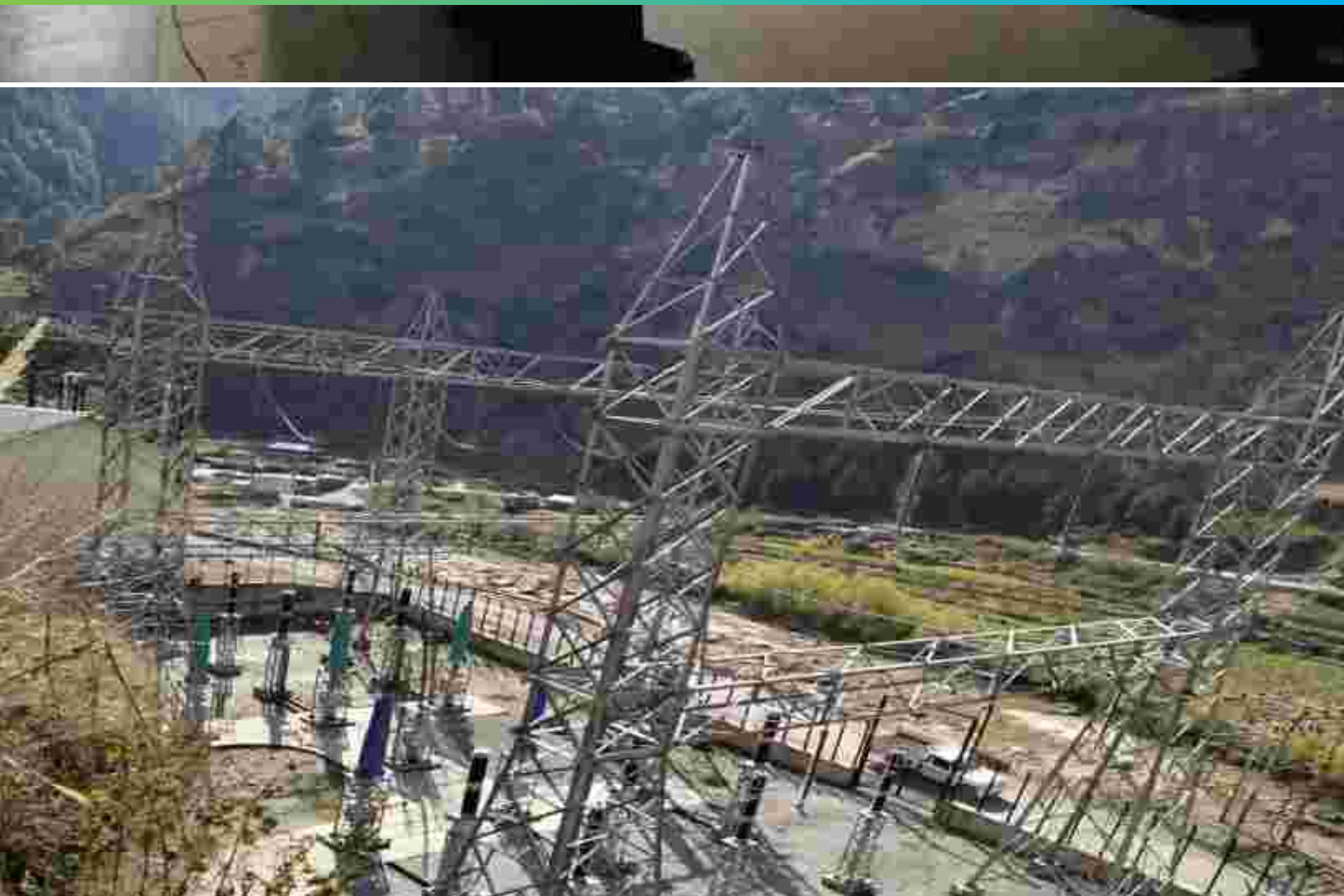
Pot Head Yard, Sawra Kuddu HEP (111 MW) PH Package
