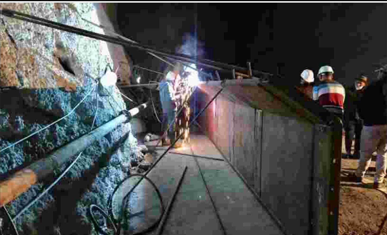
Face-V Kerb Concreting, Shongtong Karcham HEP (450 MW)
