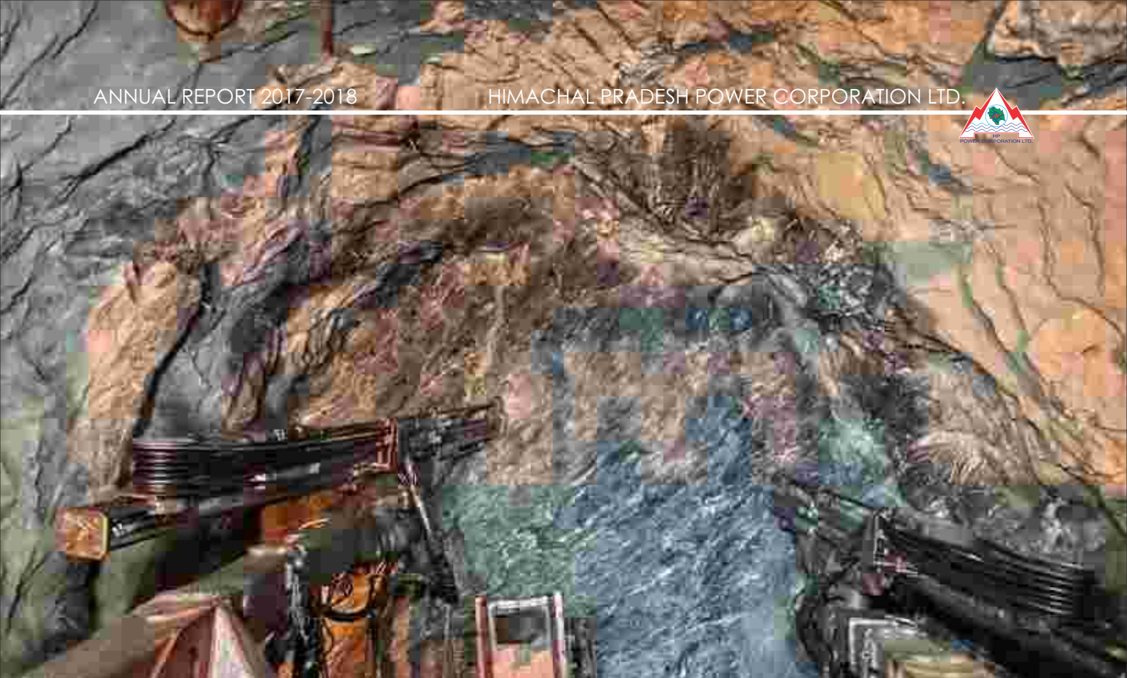
Adit to SFT Excavation in Progress, Shongtong Karcham HEP (450 MW)
