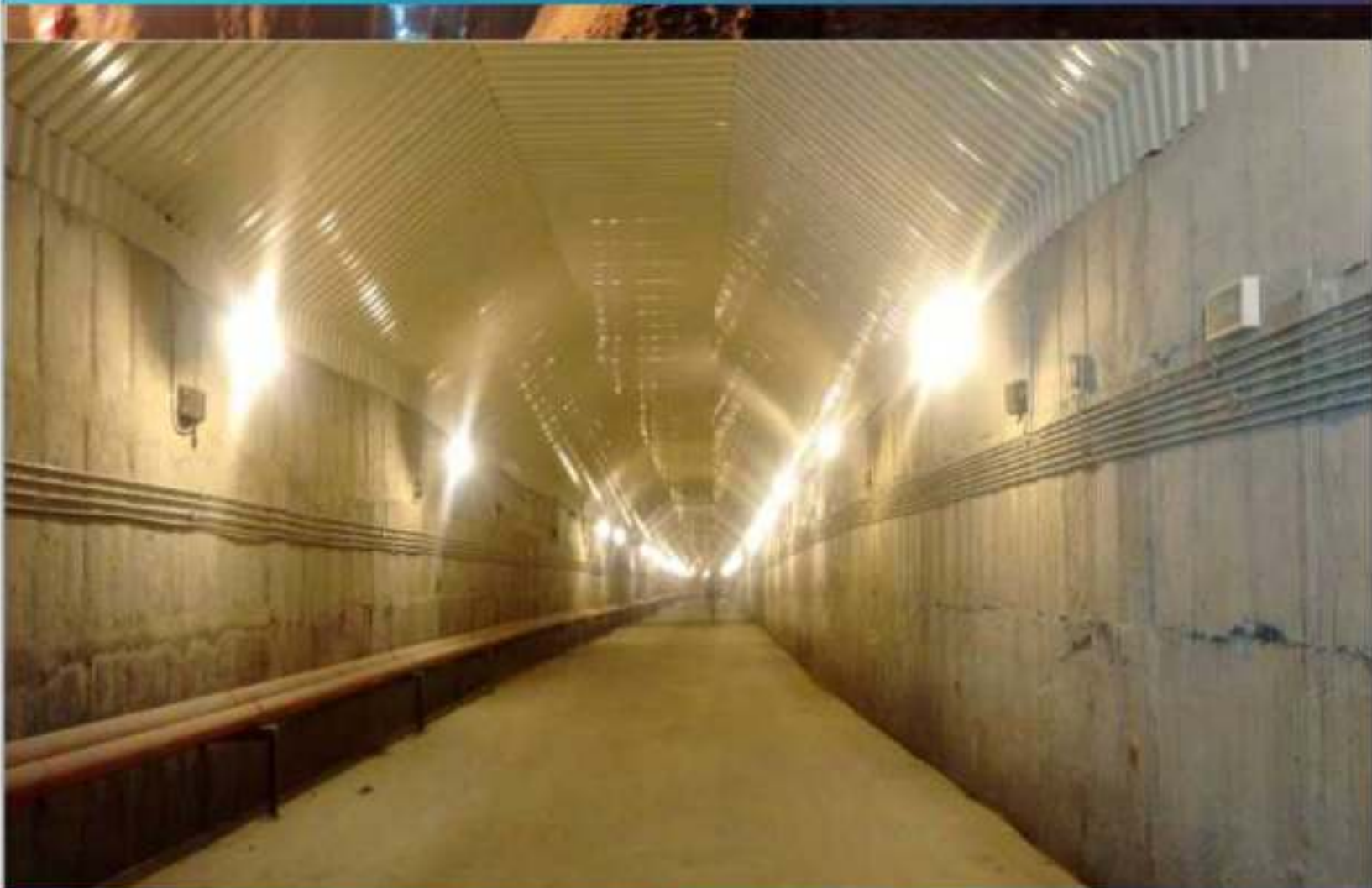
Main access Tunnel of Sainj HEP (100 MW)
