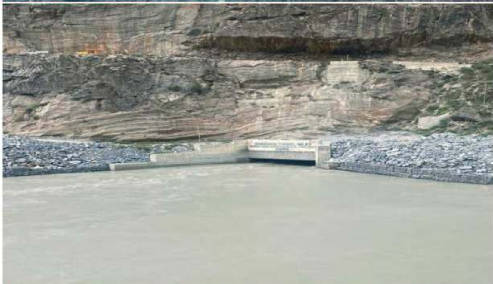
Shongtong Karchham HEP (450MW) - Diversion Tunnel Inlet
