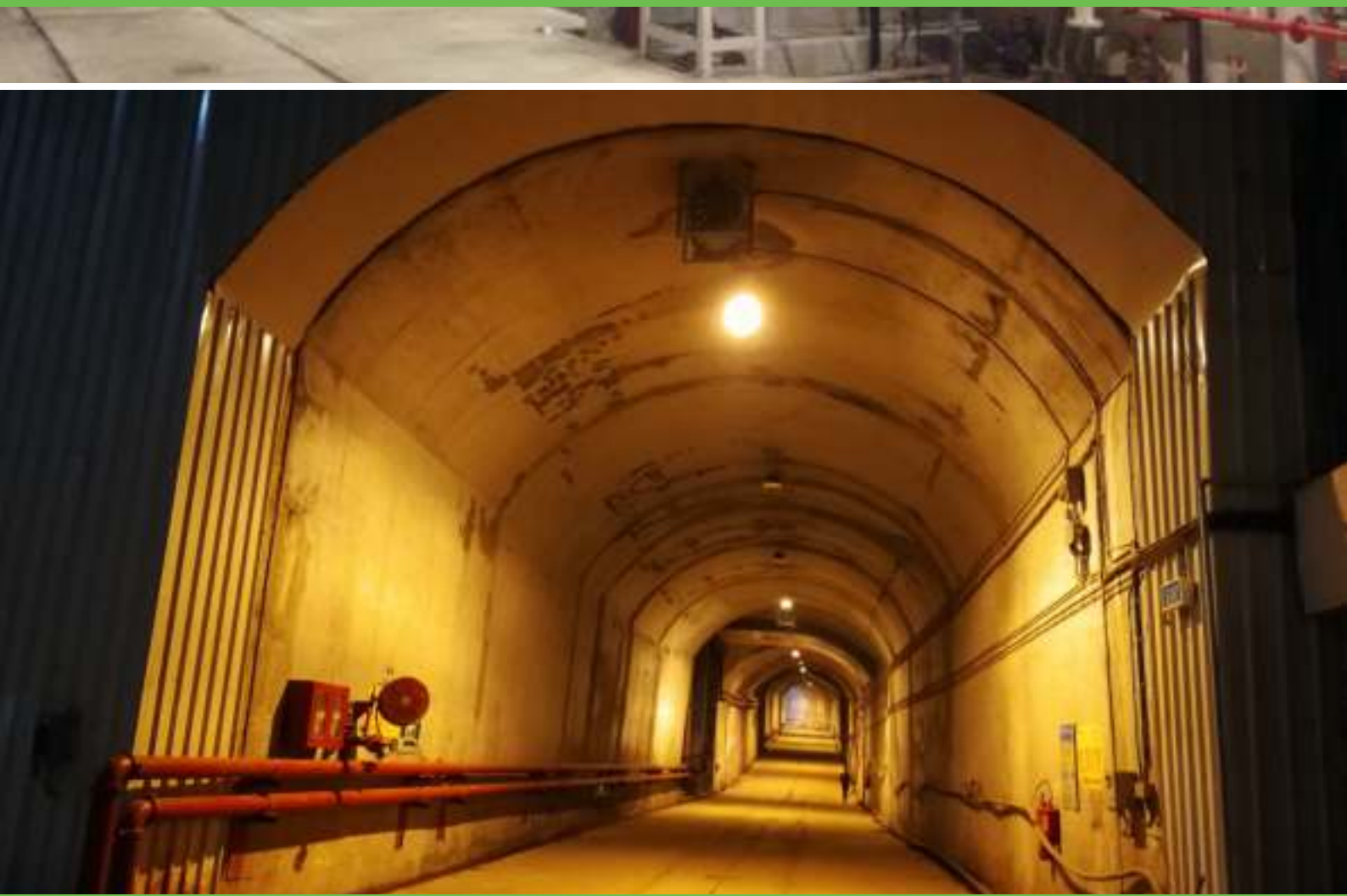
Fire Fighting Pipeline along MAT, Sawra Kuddu HEP (111 MW)
