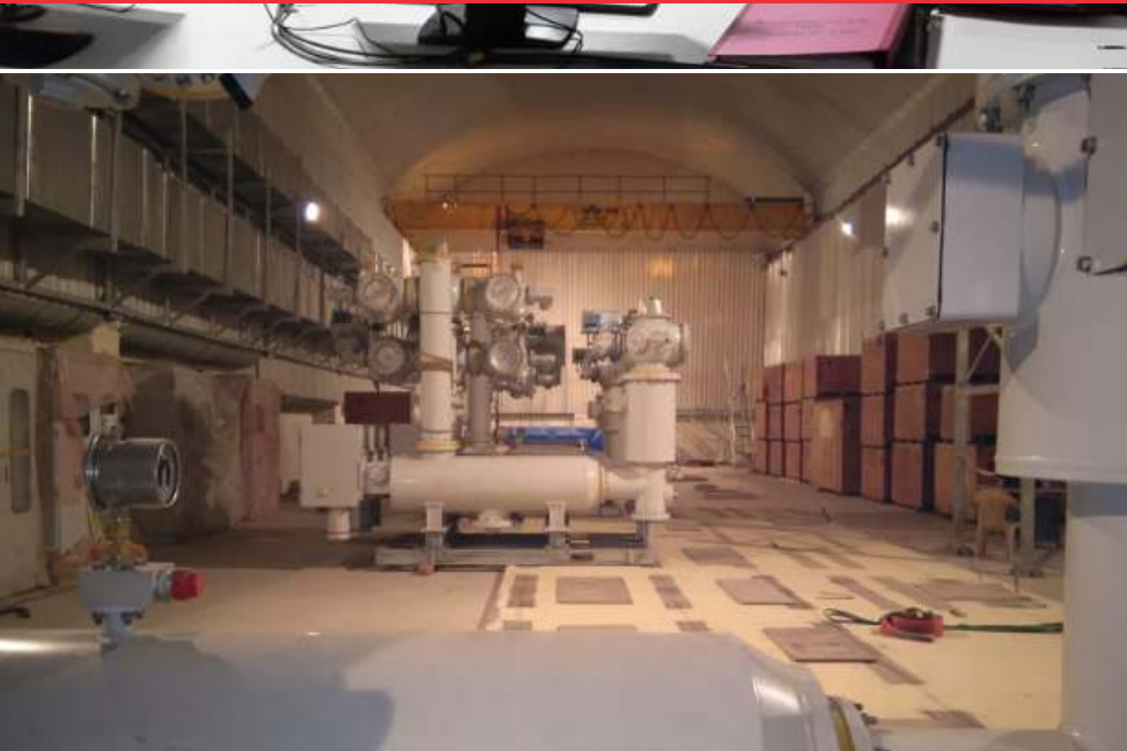
GIS Hall, Sainj HEP (100 MW)
