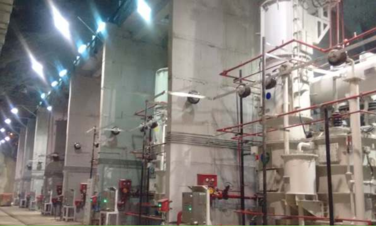
Generator Hall, Sainj HEP (100 MW)
