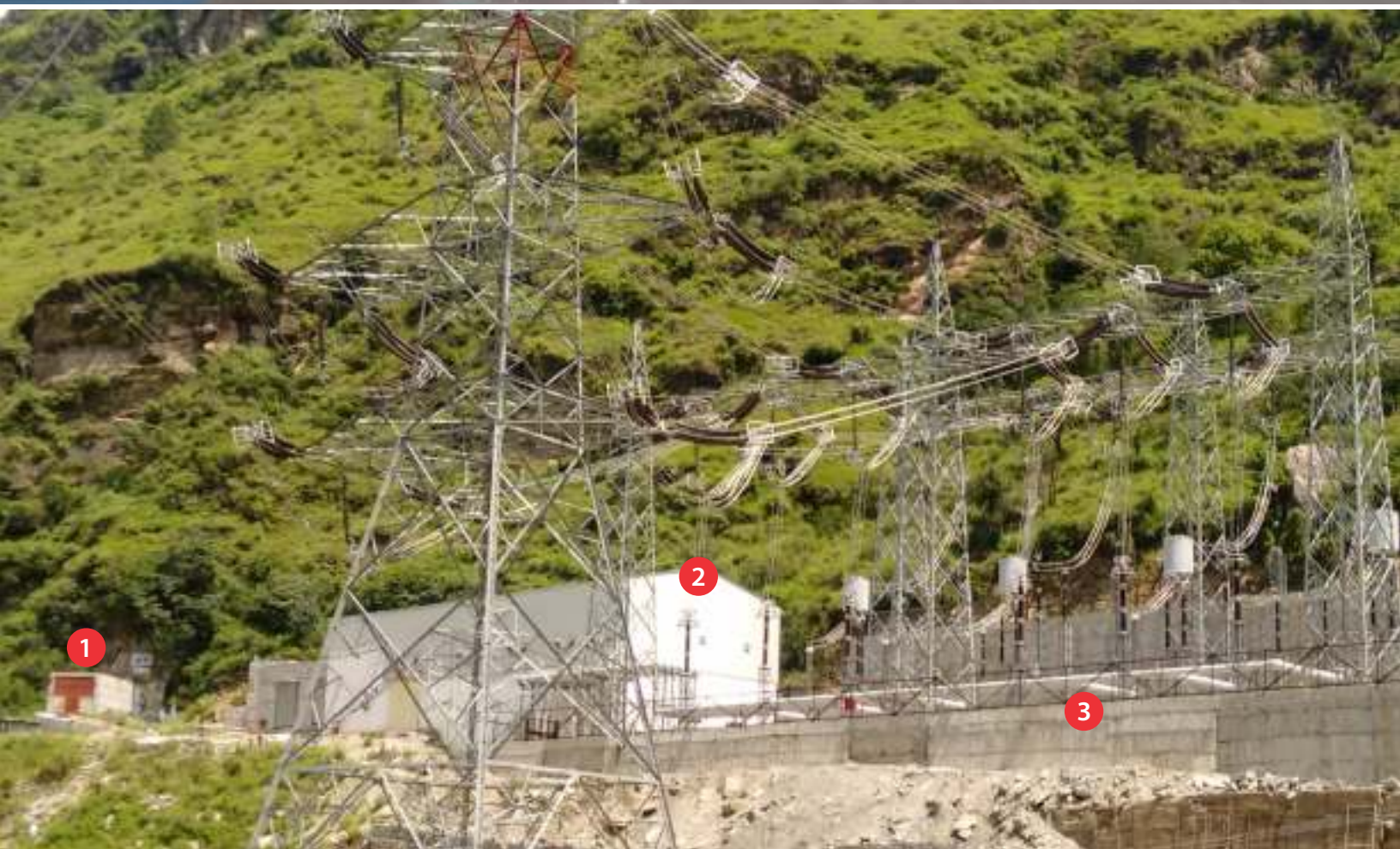
1-CVT Portal, 2-GIS Building, 3-Pothead Yard , Sainj HEP (100 MW)
