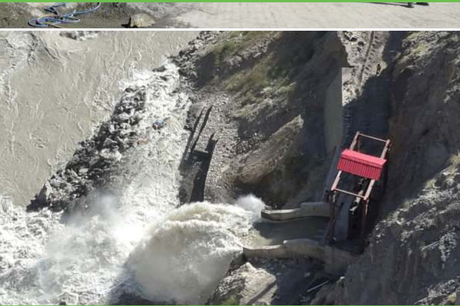
Tail Race Tunnel Outfall, Kashang HEP Stage-I (65 MW)
