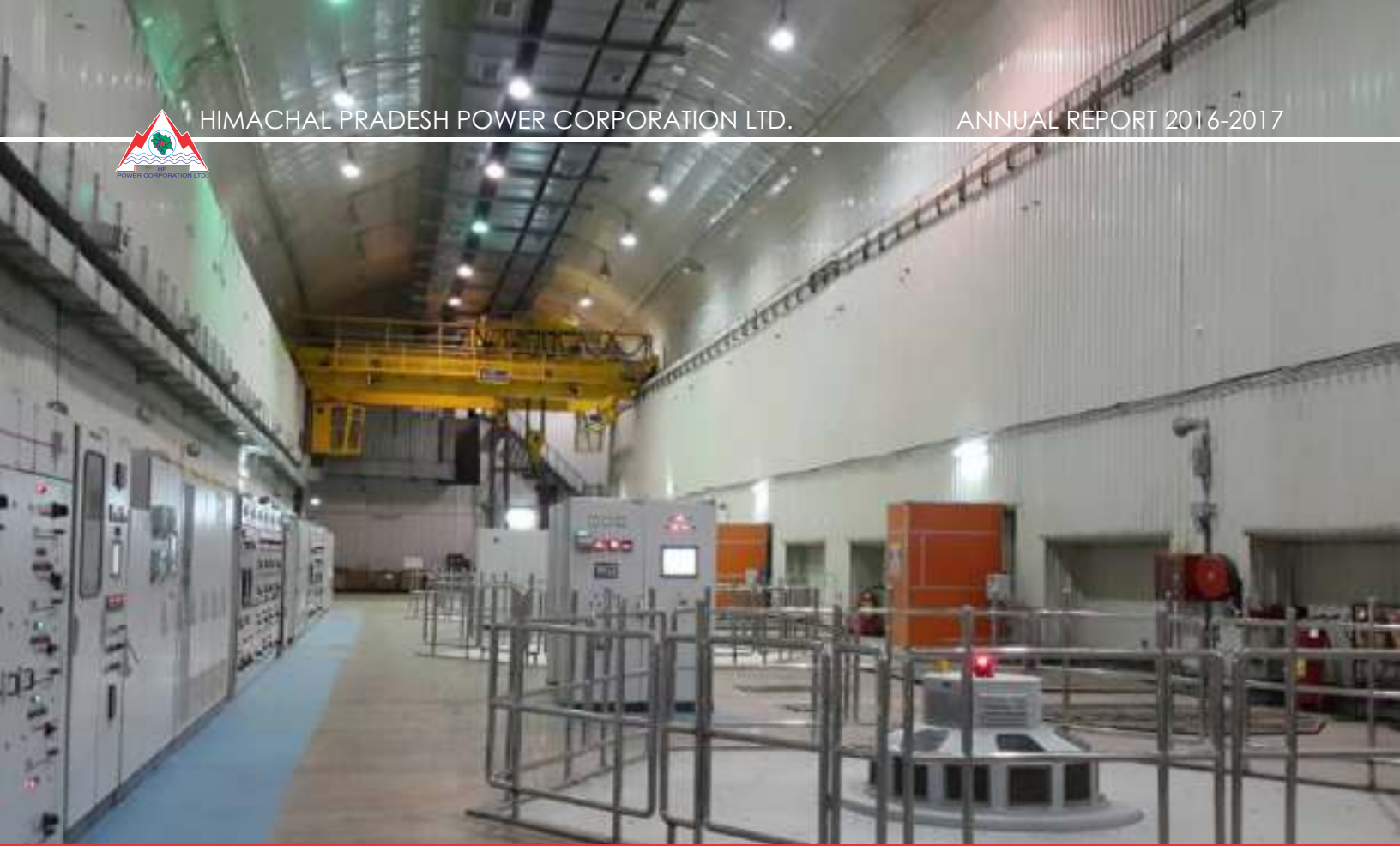
Machine Hall, Kashang HEP (65 MW)
