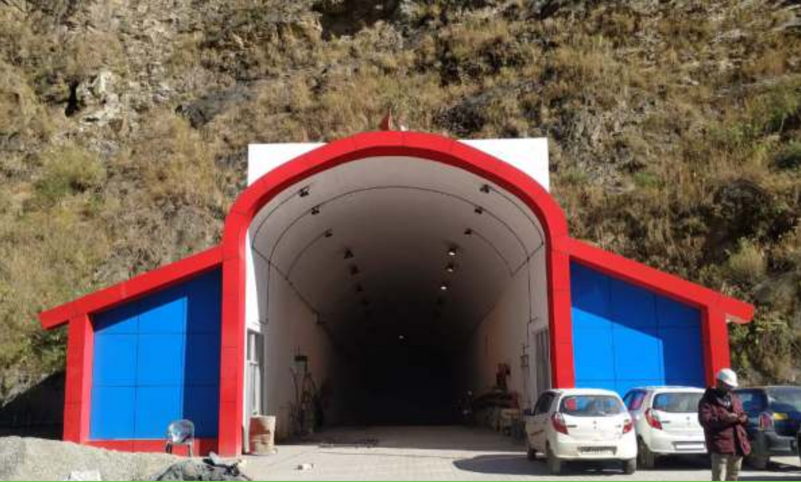
MAT Portal, Power House, Sawra Kuddu HEP (111 MW)
