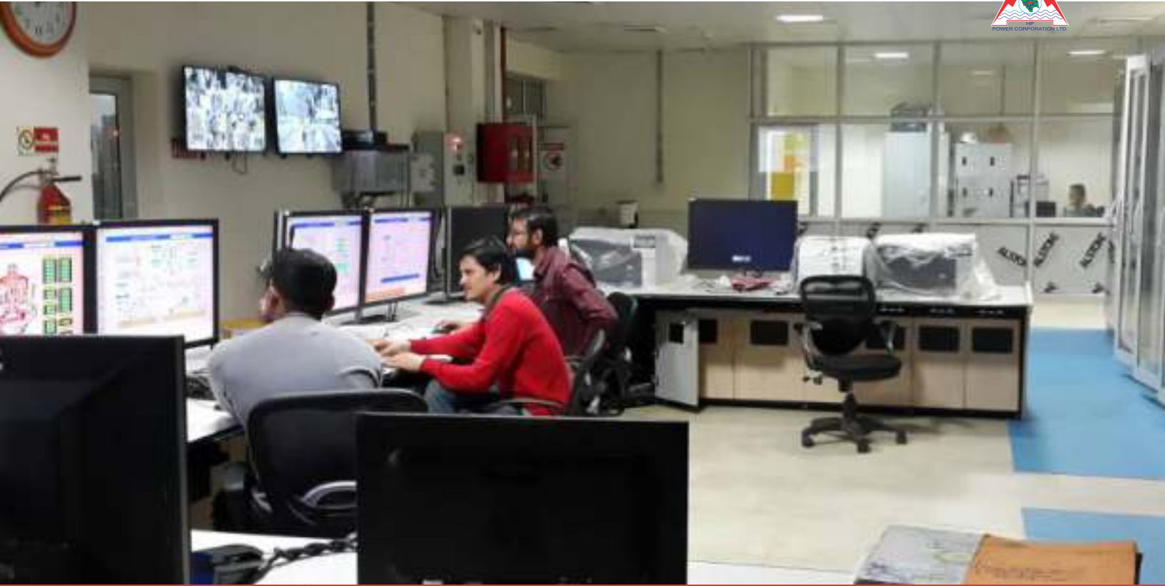
Power House Control Room, Sainj HEP (100 MW)
