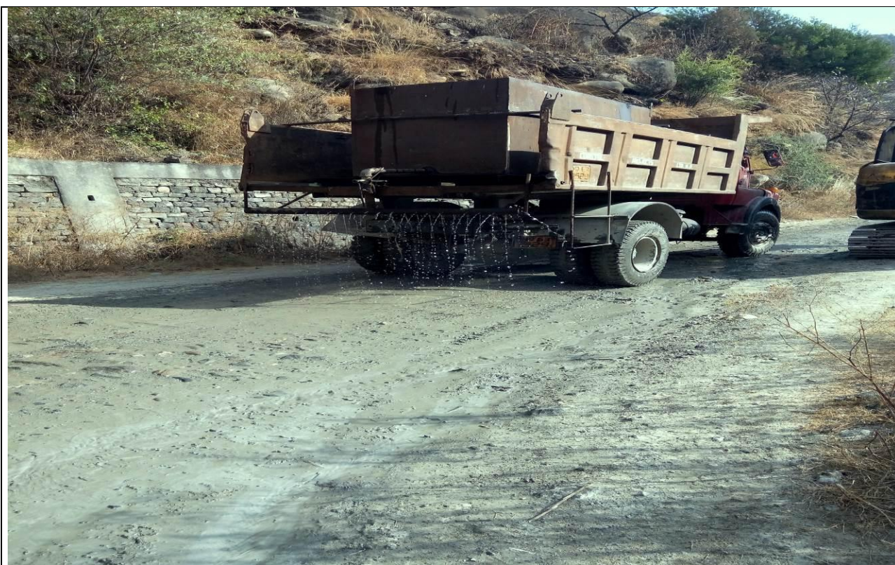
Water Sprinkling On the Project Roads
