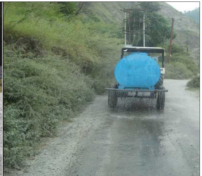
Water Sprinkling On the Project Roads (Snail)
