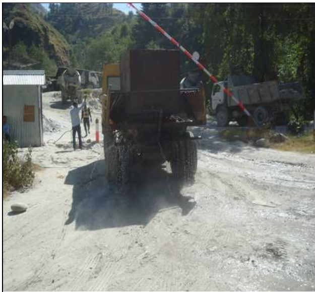
Water Sprinkling On the Project Roads (Hatkoti)
