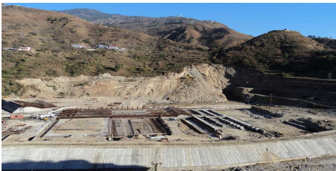
View of the submergence area and proposed barrage site
