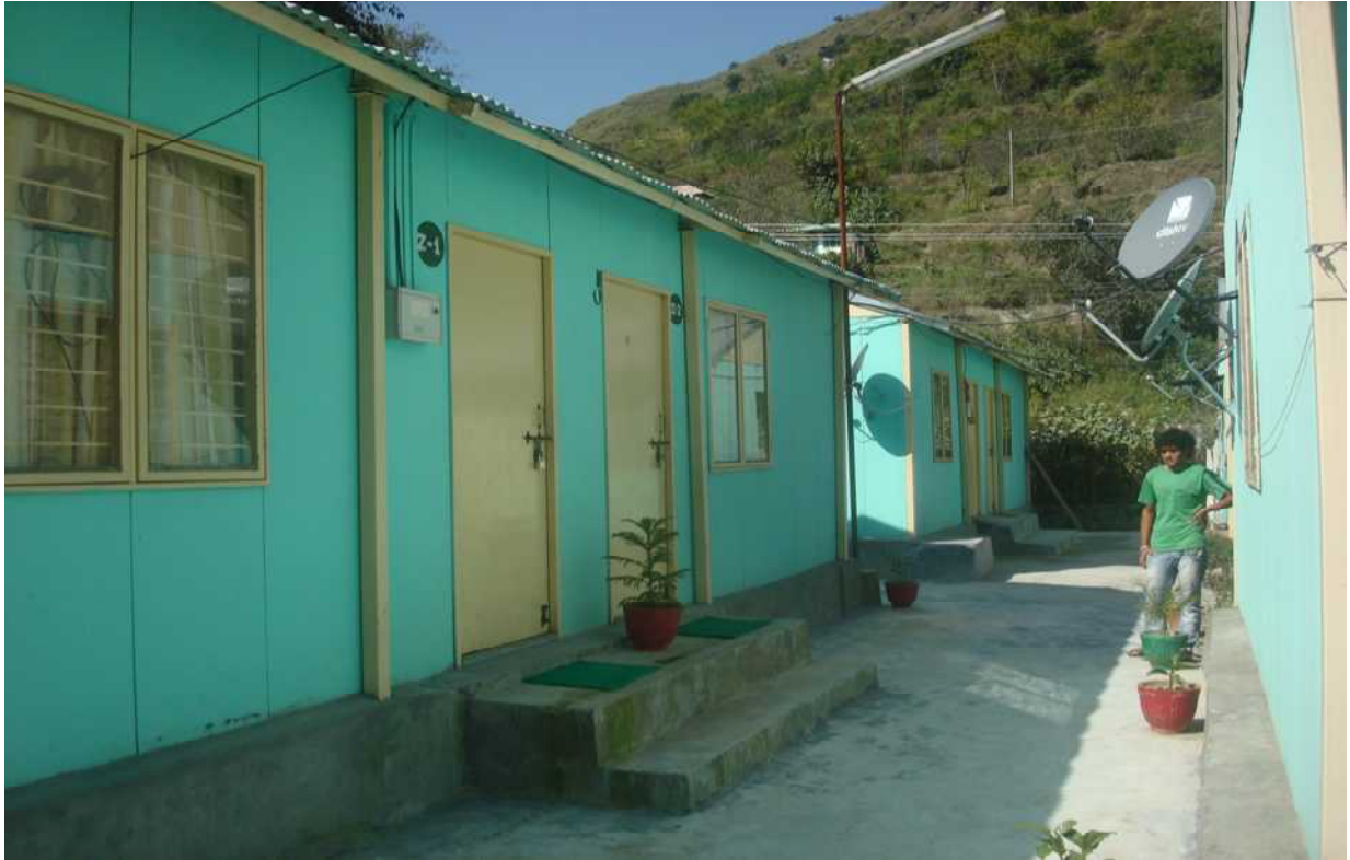
Labour colony complex near Hatkoti {also shows satellite TV antennae set up for labour}
