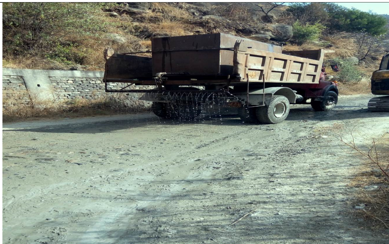
Water Sprinkling On the Project Roads
