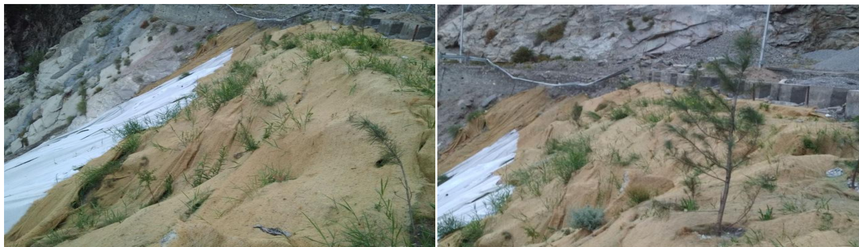
Reclamation of Dumping site at Power House of IKHEP with Geo -Tech ,Net Green blanket
