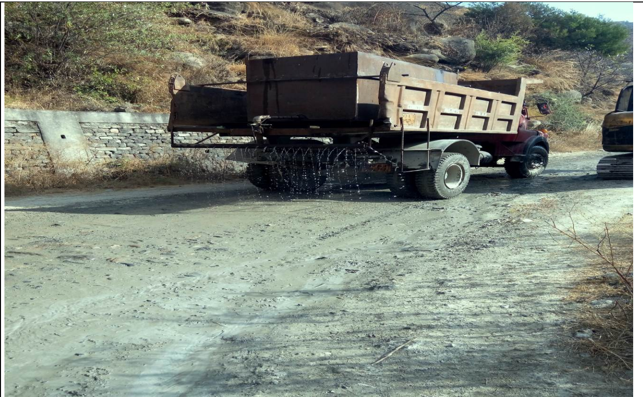
Water Sprinkling On the Project Roads
