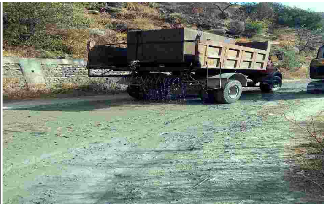
Water Sprinkling On the Project Roads
