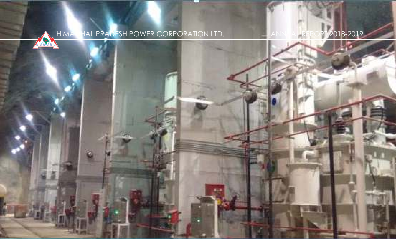
Generator Hall Sainj Hydro Electric Project (100 MW)
