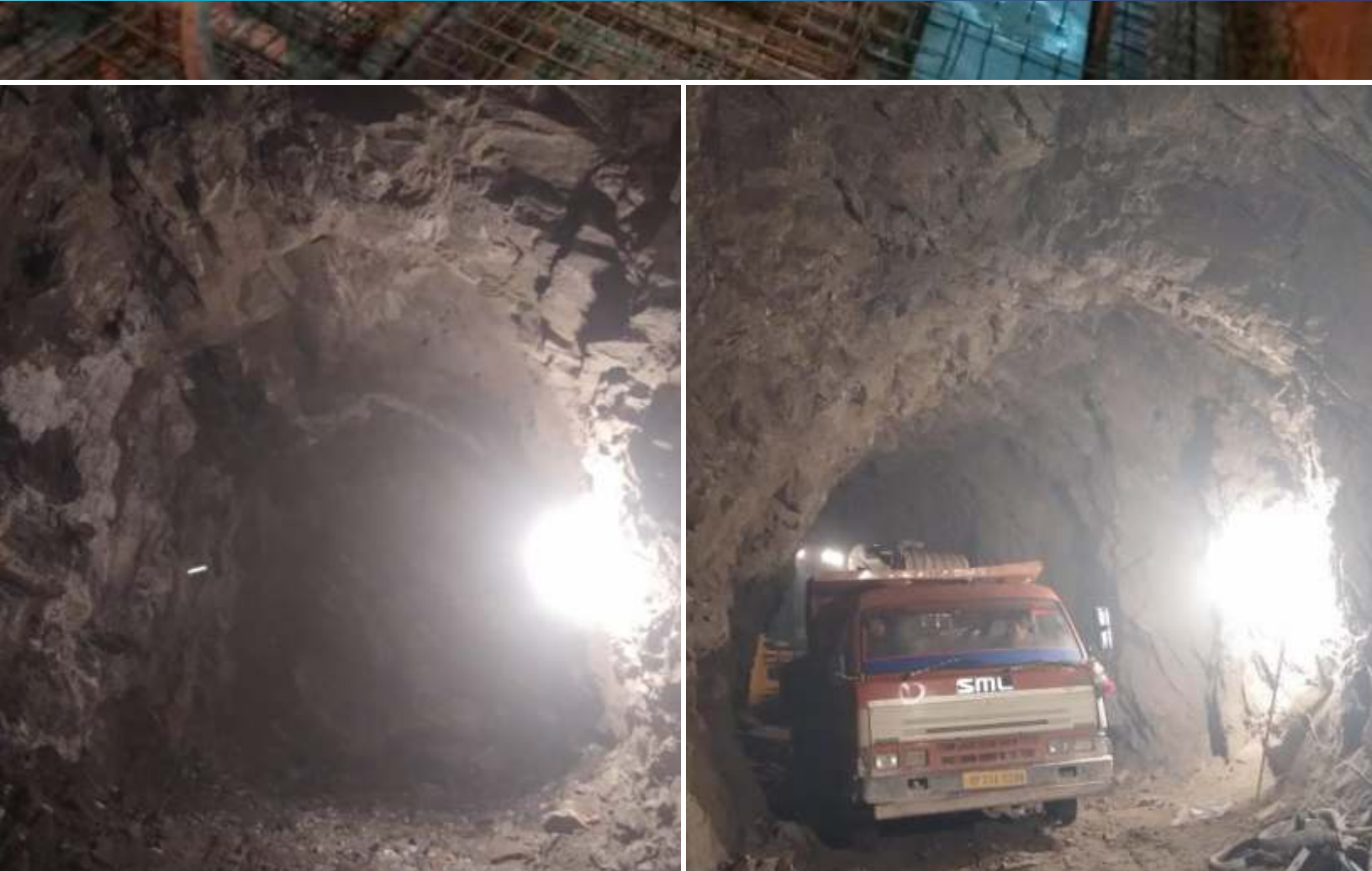
Approach Tunnel to GOC (Link Tunnel) - Excavation in progress, Integrated Kashang HEP Stage II & III
