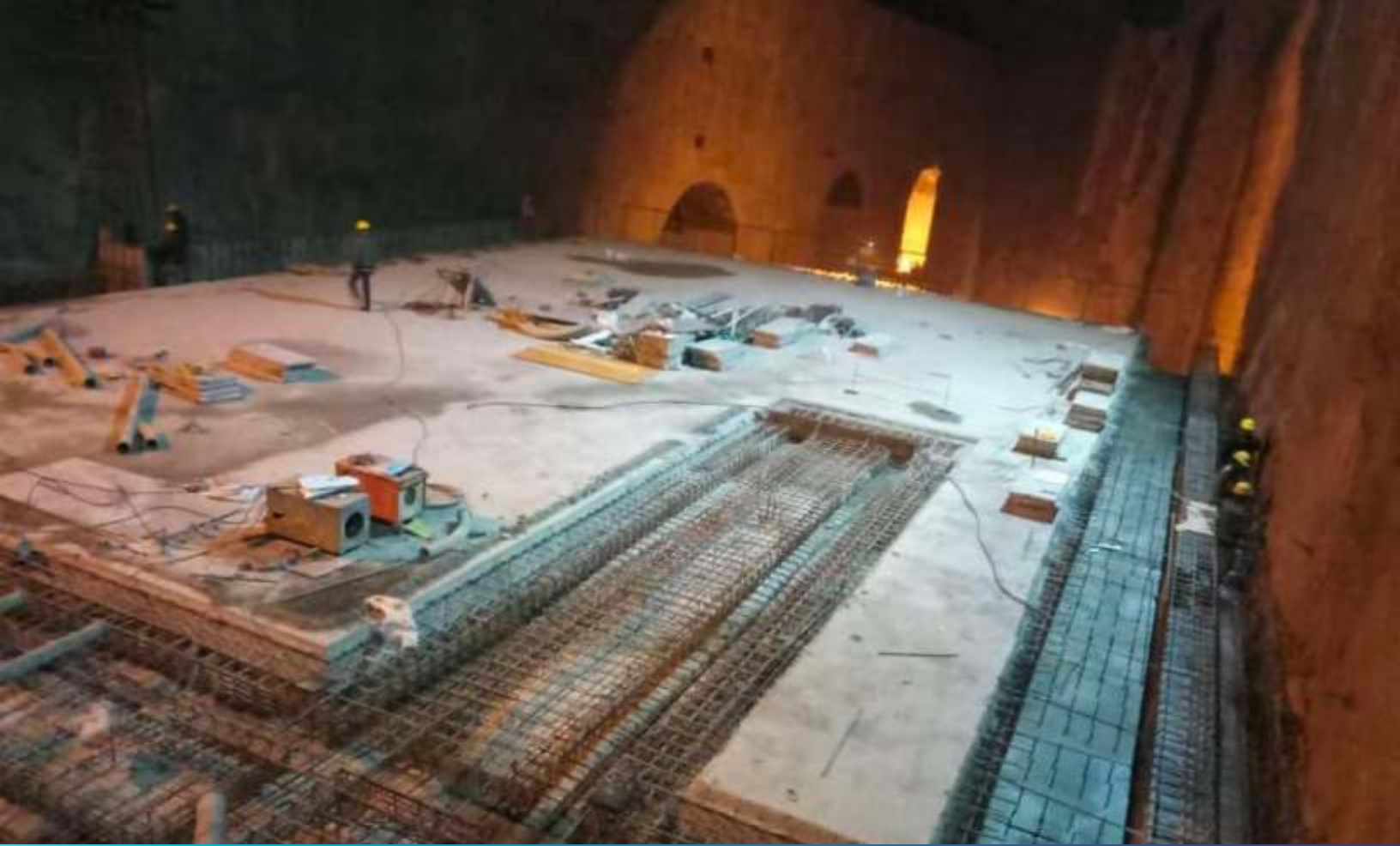
Service Bay Concreting in Progress, Shongtong Karcham HEP
