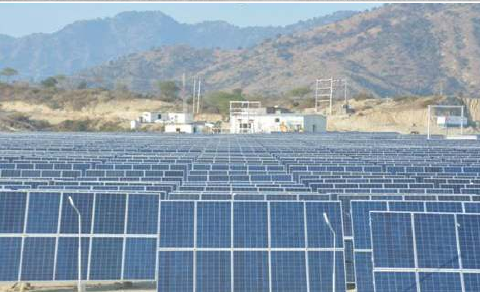
Bera Dol Solar Power Project (5 MW)
