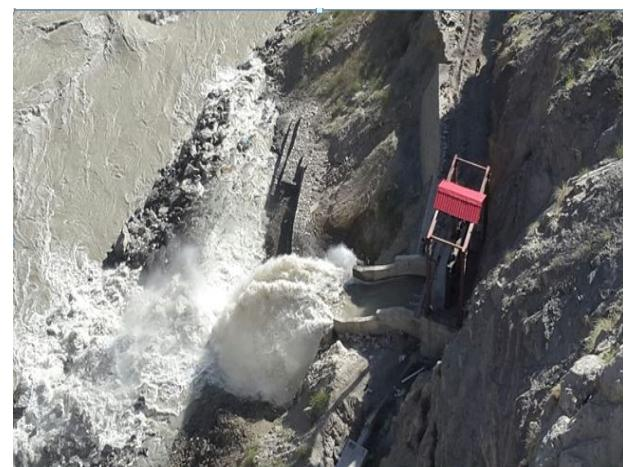
Tail Race Tunnel Outfall Kashang Hydro Electric Project (65 MW)
